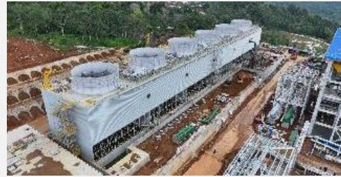
Construction LMB Power Plant
